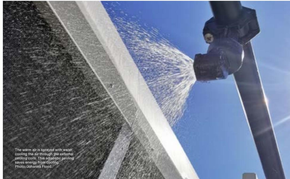
The warm air is sprayed with water, cooling the air through the external cooling coils. This adiabatic cooling saves energy from cooling.
